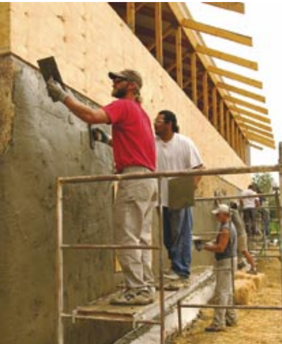
Teaching by example: Construction Program Director Mike Kelly and construction trades student Dave LeDoux applying stucco to the ERC walls.
