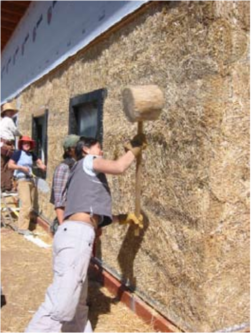
Selena Murphy uses the “eliminator” to plumb up a wall.
